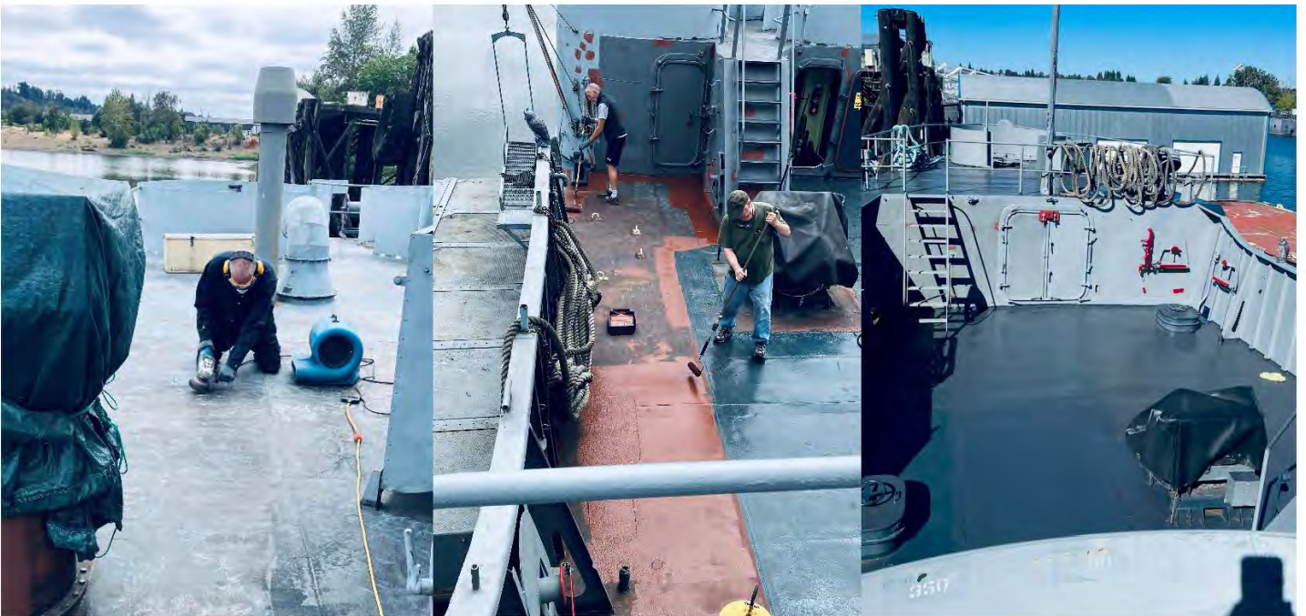
Many hours of wire wheeling on the decks, painting the well deck. Now it's looking good!
