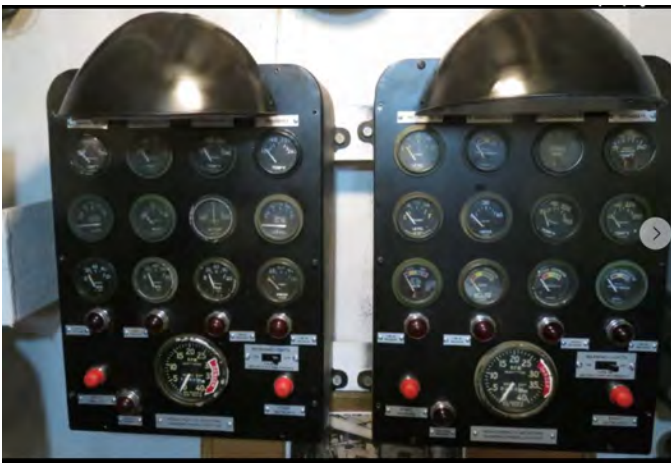
Engine room gauge panels per original spec By Dennis Weehunt.
