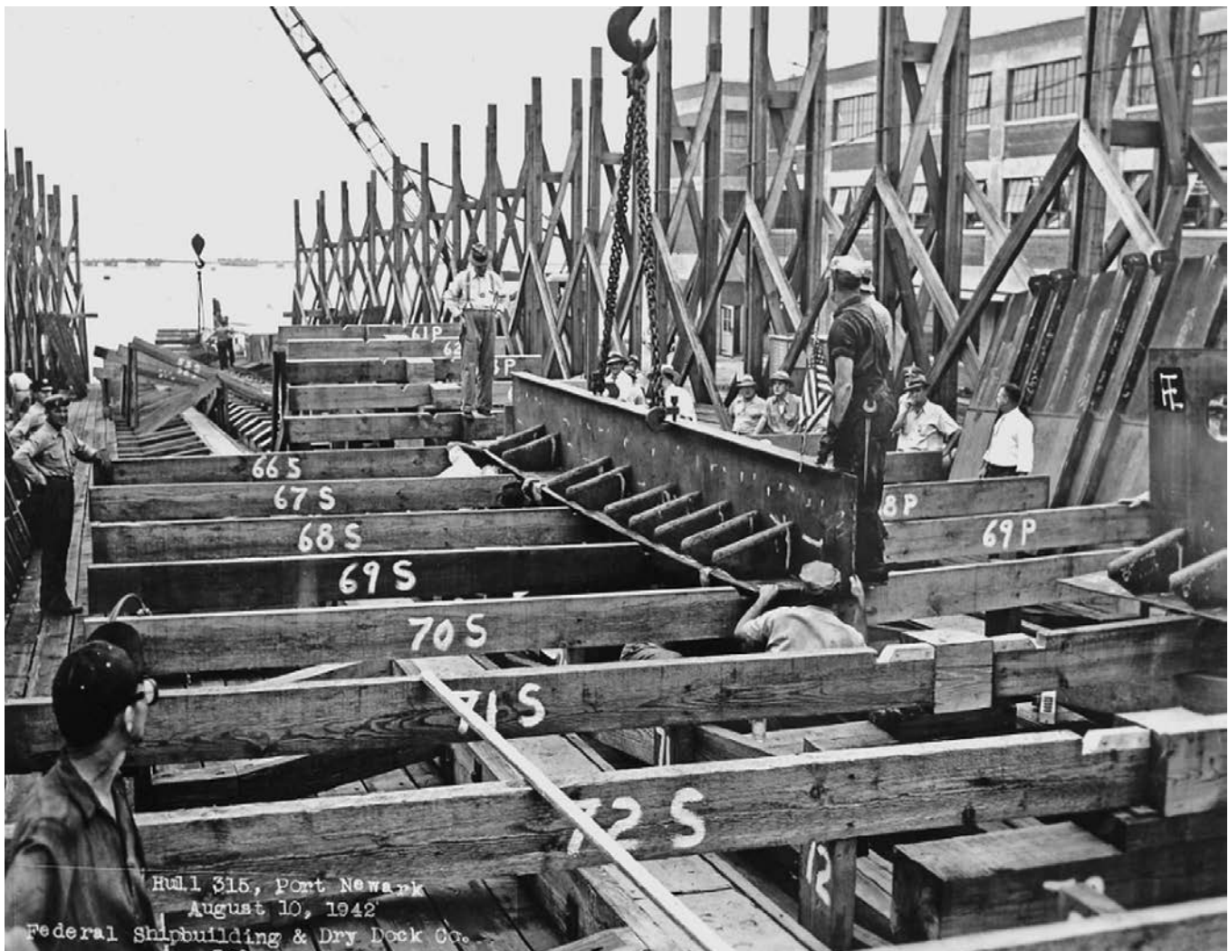
The keel is laid for LCI(L) 315 at Port Newark, New Jersey, on 10 August 1942. This was a construction site for Federal Shipbuilding & Drydock Company, a major builder of LCIs during the war. Over half the Navy would become amphibious. NARA 19LCM-LCI(L) 315.
