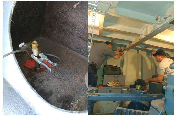
Stuffing tube for stern running light
