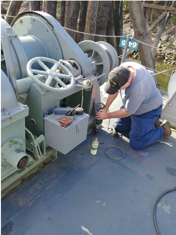
Sound Powered Phone Box & system install
