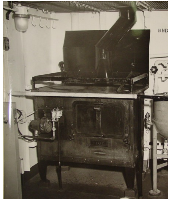
The Webbperfection Model 120. The stove, which burned diesel fuel, WP-120's had one top burner and an oven. The LCI-713 had two, side by side.
