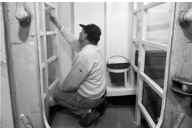
The final touches of paint in the Magazine!
