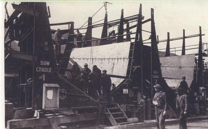
LCI'S ARE BUILT in sections which later are welded together. This shows two bow sections under construction.
