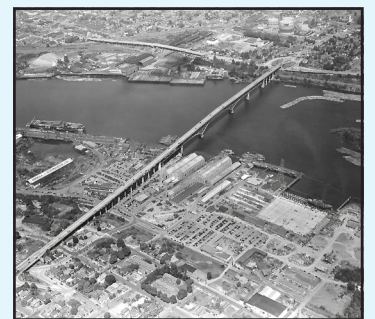
Aerial view of Commercial Iron Works straddling Ross Island Bridge, with construction ways on right side and outfitting dock on the left.
