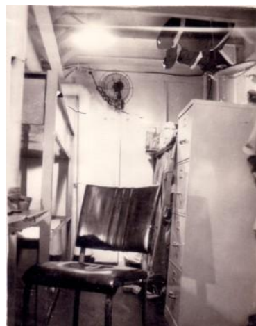
Jacket in overhead with brackets on LCI629 XO Stateroom
