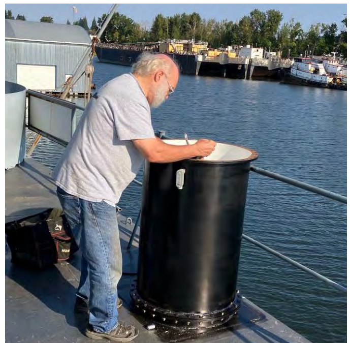
Installing wiring conduit up through the deck.
