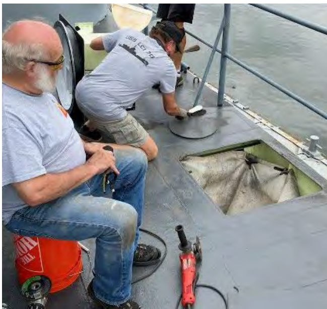
Cutting the deck to install the new fan.
