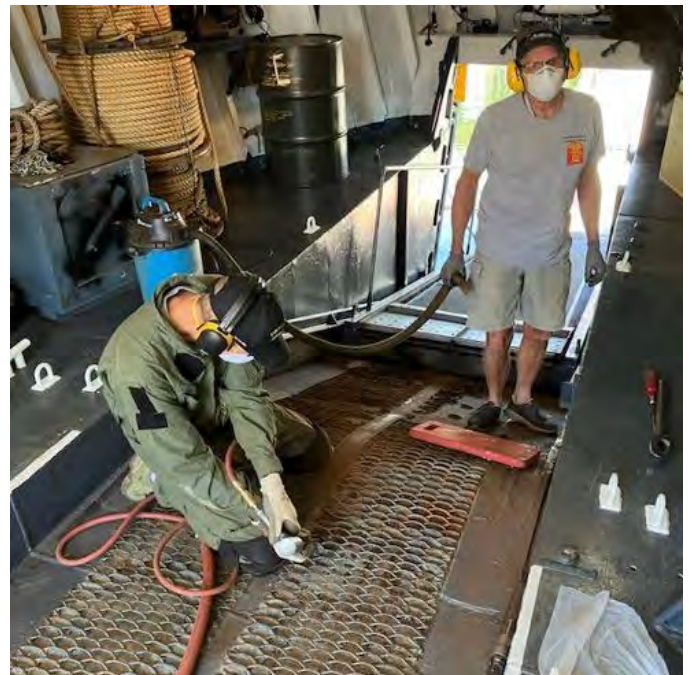
Pictured are Rick and John are busy needle gunning rust from the grating.
