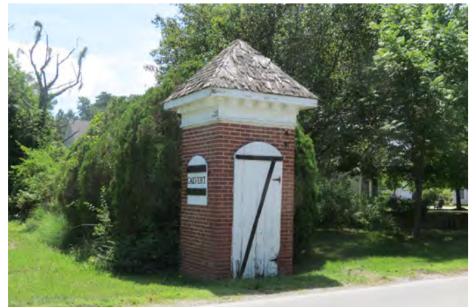
What the original Gate House looks like today.
