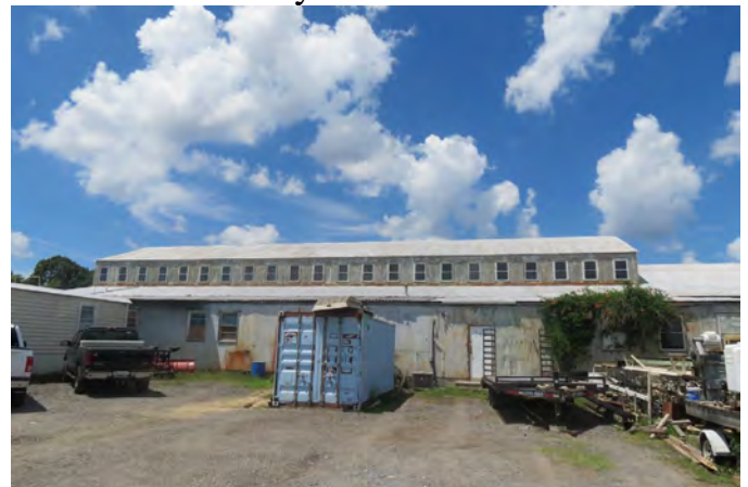
Washburn’s Boat Yard Shop Building Inside Washburn’s Shop Building. Note the Lifting Trolley / Beam tracks.
