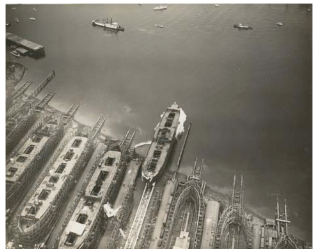
Another liberty ship hull launched. The Kaiser northwest shipyards built and launched 752 ships during WWII.
