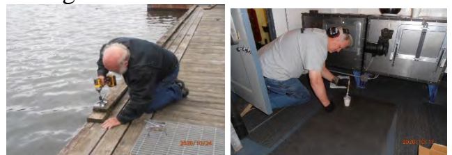
Dock repair and Galley stove rust proofing
