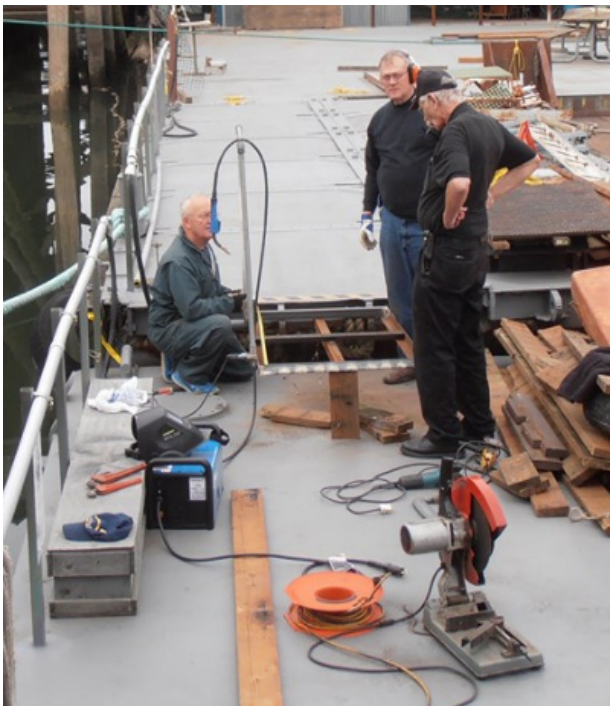
Mark, Lin and Phil installing new access ramps.
