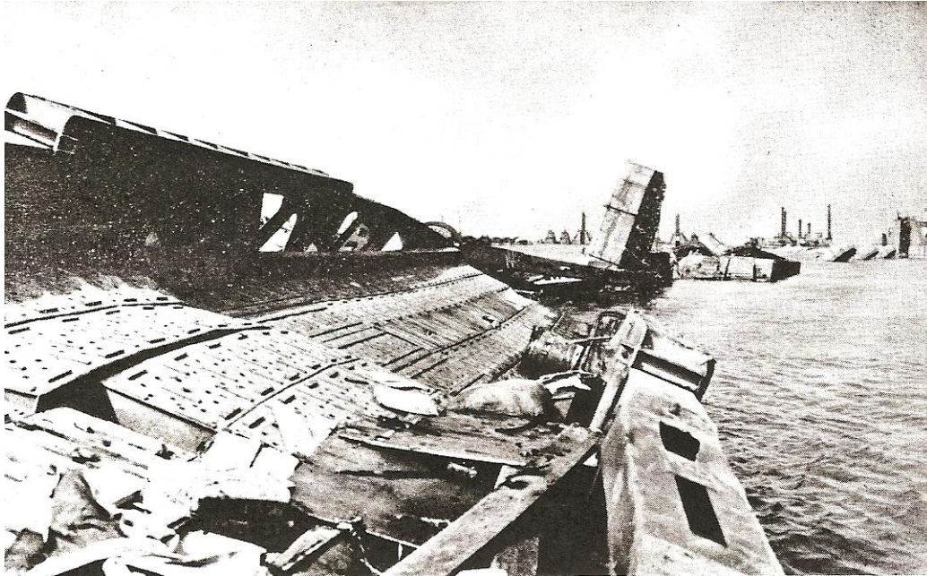
The twisted wreckage of the Whale roadway to shore. Drifting landing craft had crashed into it during the storm. (U.S. Navy photograph)
