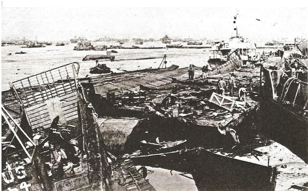
This picture at low tide after the storm shows some of the barges and landing craft that piled up against the Whale roadway. (U.S. Navy photograph)
