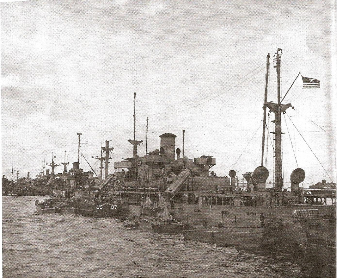
Gooseberry breakwater off Omaha Beach, formed by a line of sunken ships. Note the landing craft inside the sheltered area. (U.S. Navy photograph)
