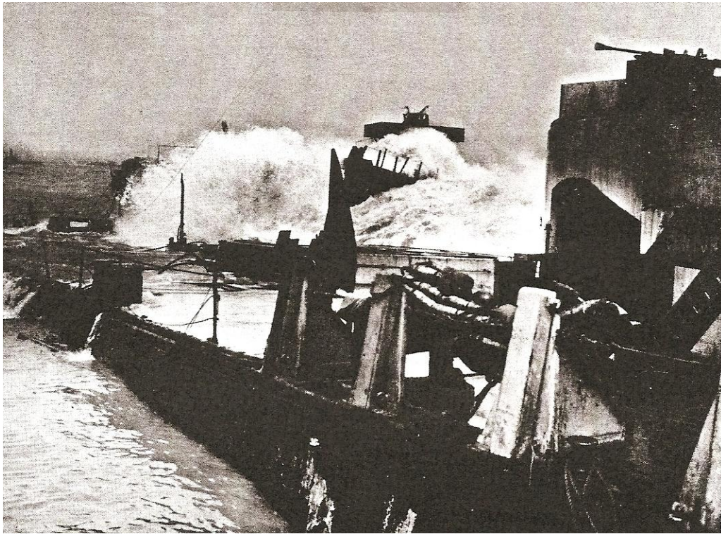
A huge storm wave breaks over the deck of the old Centurion , the outer ship at the end of the Gooseberry breakwater. (U.S. Navy photograph)
